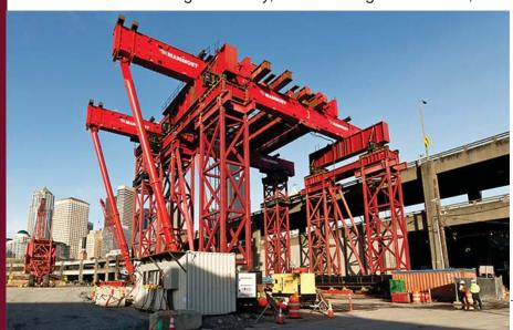
216 steel ribs and plates as added reinforcement. When completed, crews will reverse the rigging process and lower the assembly back into the shaft for reinstallation.
